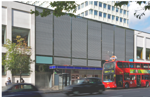
Lancaster London Hotel // Project with Neil Mathews Architects
